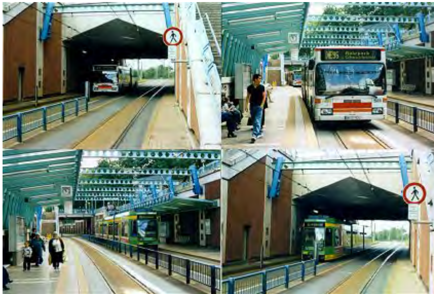
Figure 10-6 Shared Bus and Light Rail (Tram) Facilities
